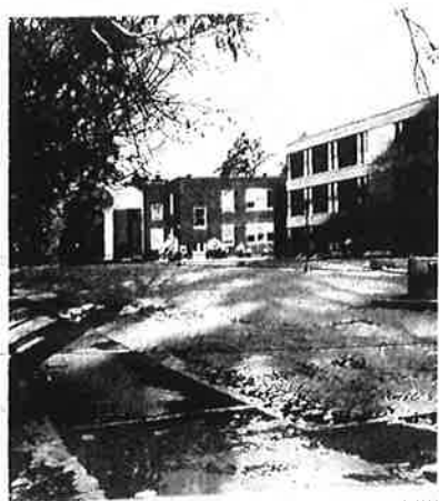
CEMENT, PLASTER, AND OLD MAIN
