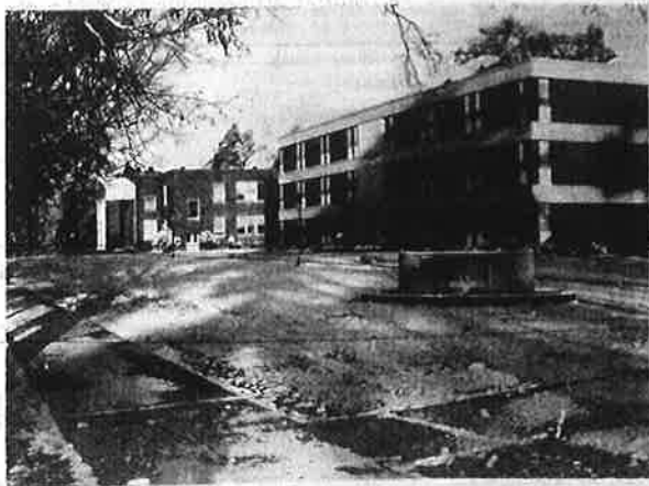
CEMENT, PLASTER, AND OLD MAIN
